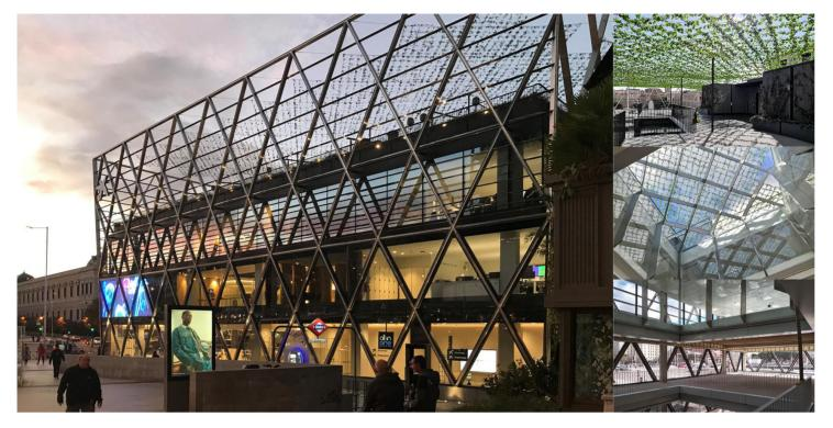
Refurbishment of the building located at Colón 1 Square. The main structure is adapted to new commercial use in three of the levels, while the rest will be offices. The project includes the opening of a large central atrium, the removal of the existing façade and the execution of a new one as a diagrid and a catenary structure that will create a garden on the roof.
